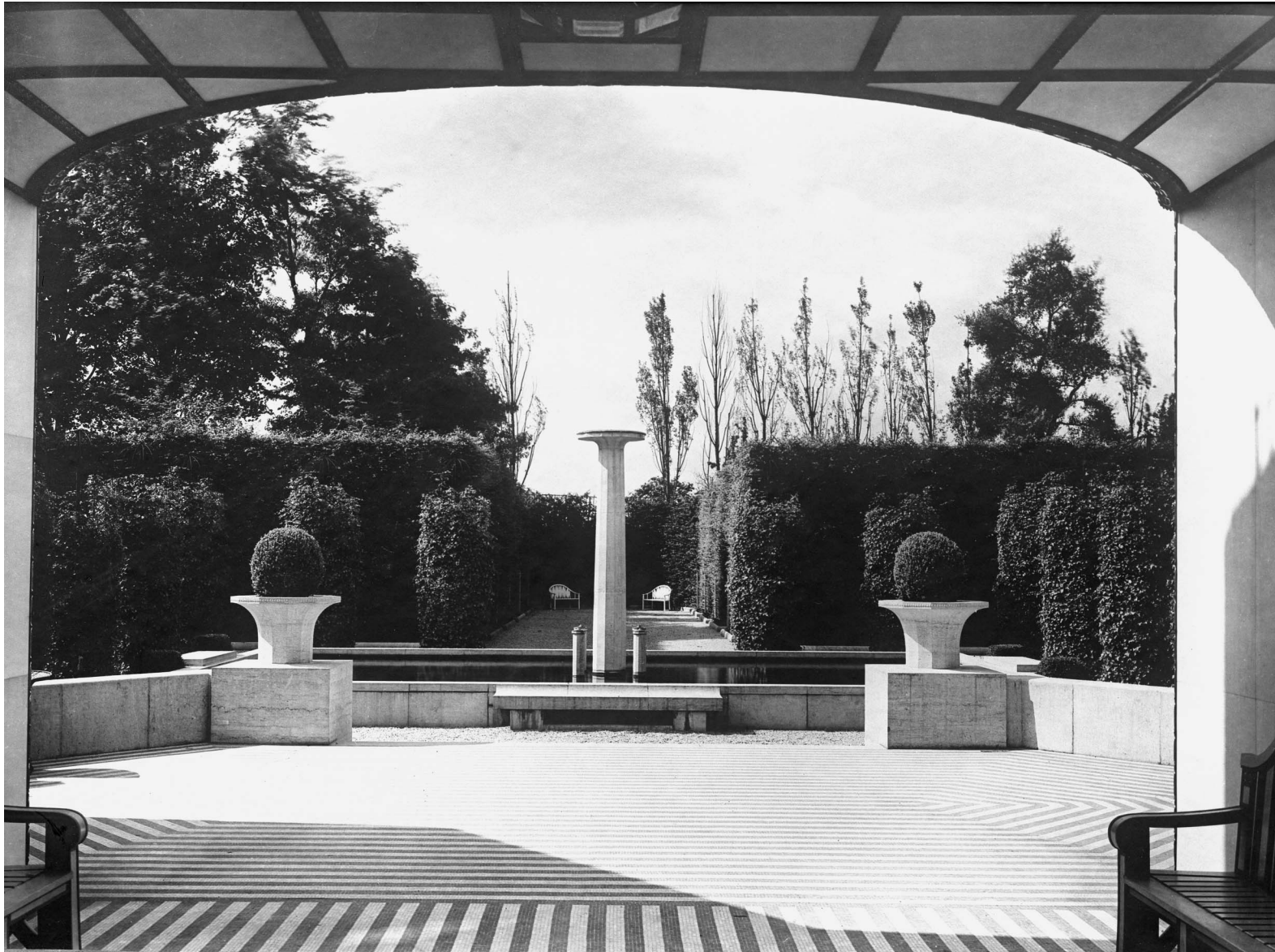
FIGURE 14. A photograph taken around 1914 shows the completed project from nearly the same viewpoint as Figure 13 (© Bildarchiv Foto Marburg, Inv. 620.288).
