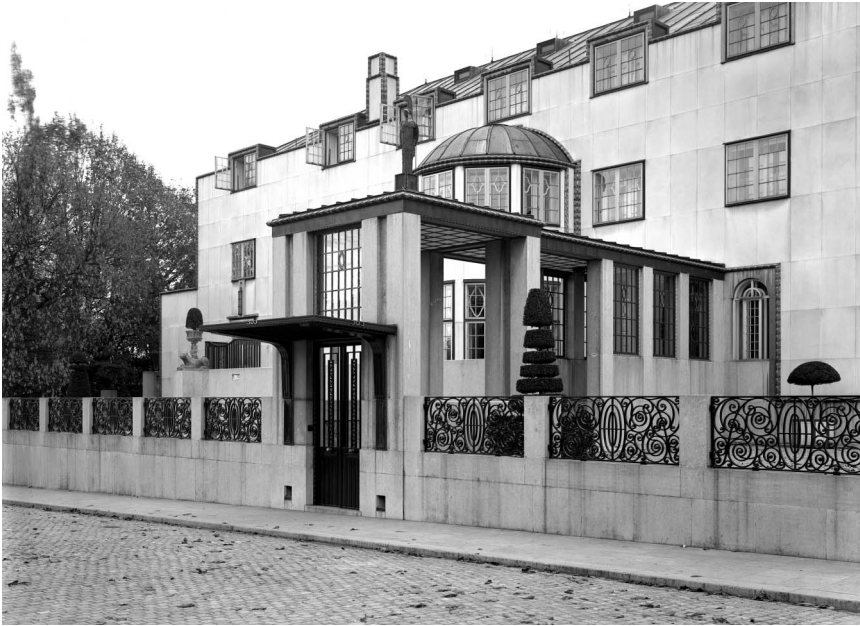
FIGURE 16. The transitional spaces between outside and inside are very important in Hoffmann's architecture and have been carefully designed (© Bildarchiv Foto Marburg, Inv. 604.445).
