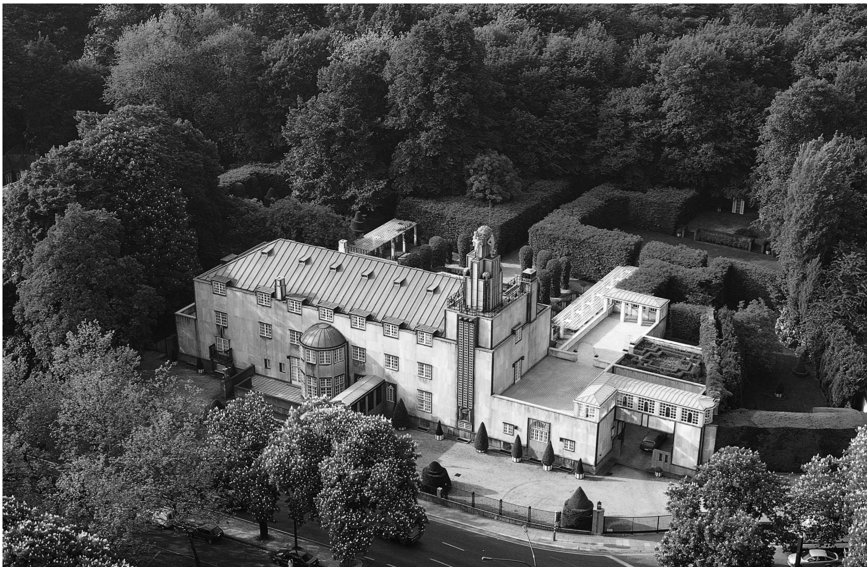
FIGURE 6. Bird's-eye view of the ensemble — the property adjacent to the servant's wing was bought in 1954 and added to the original garden (Photograph: Wim Robberechts).
